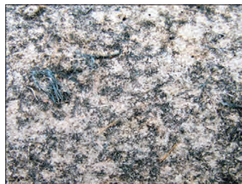
Asbestos cement sheet garage in poor condition
