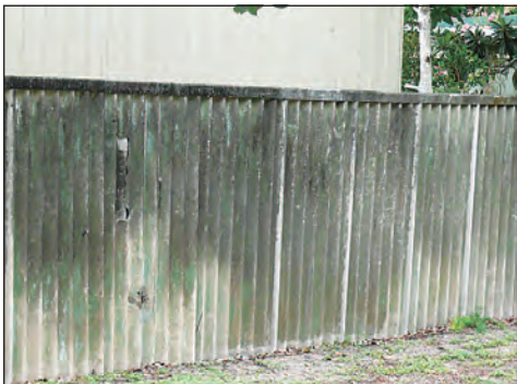
Corrugated Asbestos cement sheet fence
