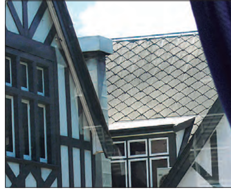
Asbestos Cement Roof shingles
