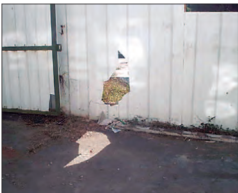
Profiled Asbestos Cement sheet
