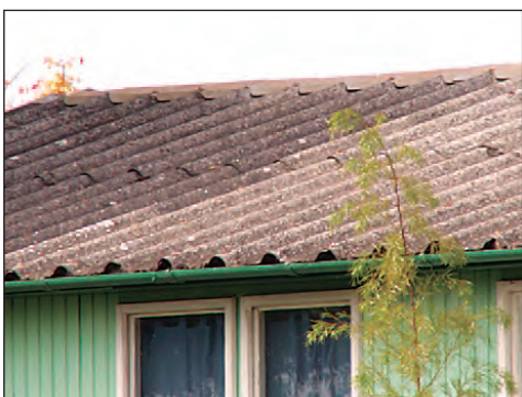
Profiled Asbestos Cement sheet
