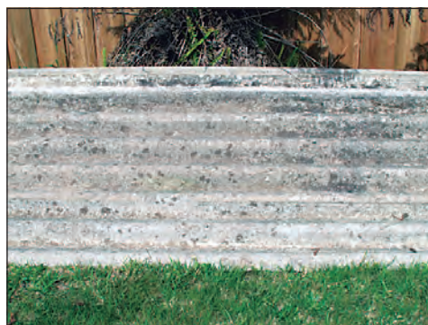
Simulated brick cladding asbestos cement
