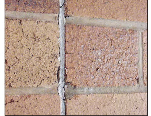
Asbestos joint sealant
