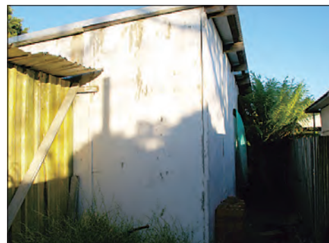
Asbestos cement sheet garage in poor condition
