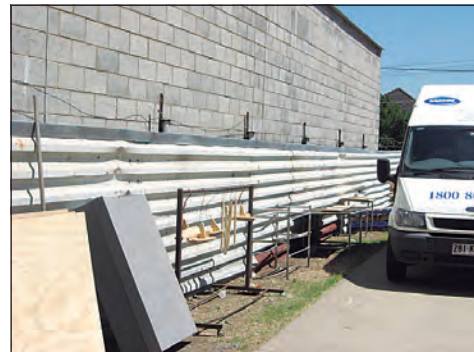
Galbestos sheeting being used as fencing
