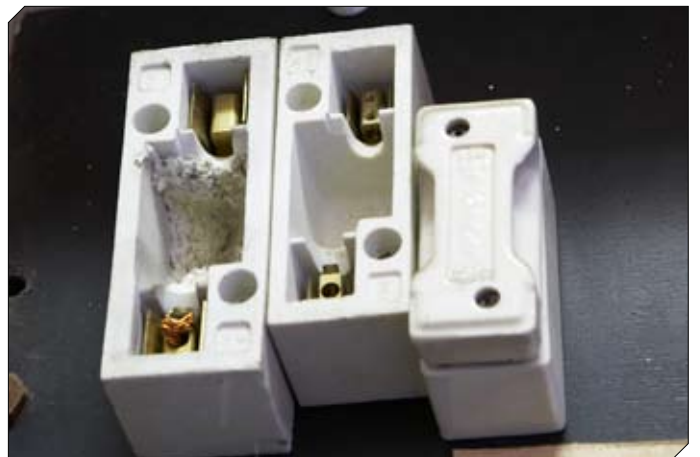
Figure 17: Friable asbestos insulation in an electrical fuse housing.
