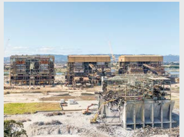
Power Block & Slot bunker 17 March 2021
