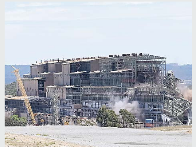
Boiler House Unit 7 Coming Down
