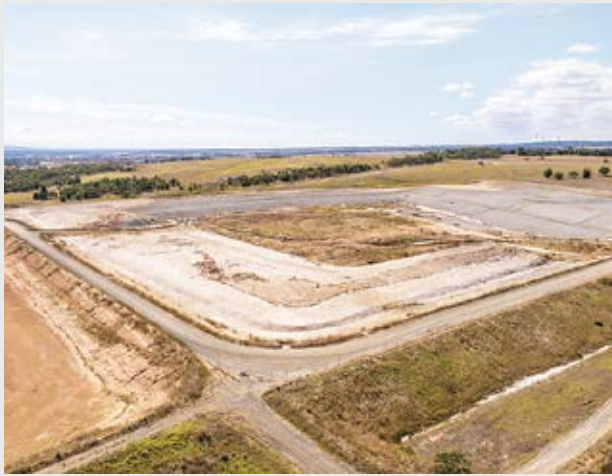
Asbestos Cell 17 March 096
