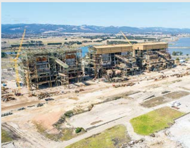
Slot Bunker and Power Block 17 March 2021
