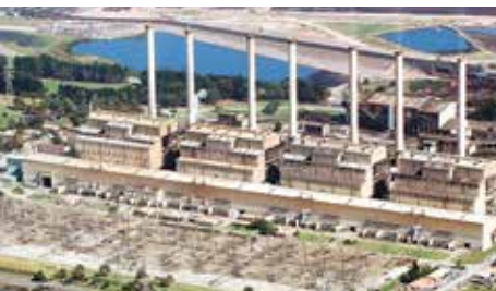
Hazelwood Power Station
