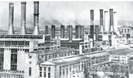
Yallourn Power Station
